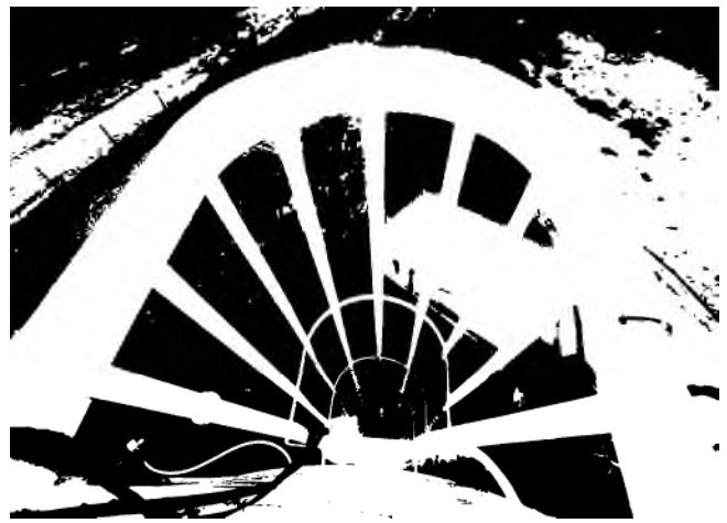
Top of safety cage
